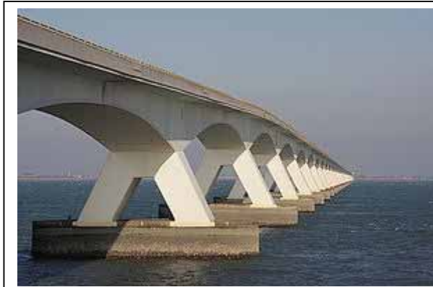
The Zeeland bridge
